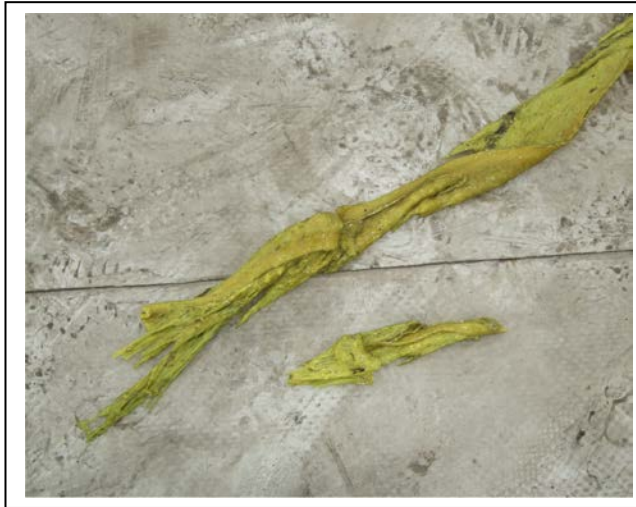
Figure 10 – Melted parapet lighting detail
