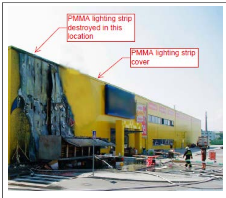
Figure 9 – Lighting detail at parapet
